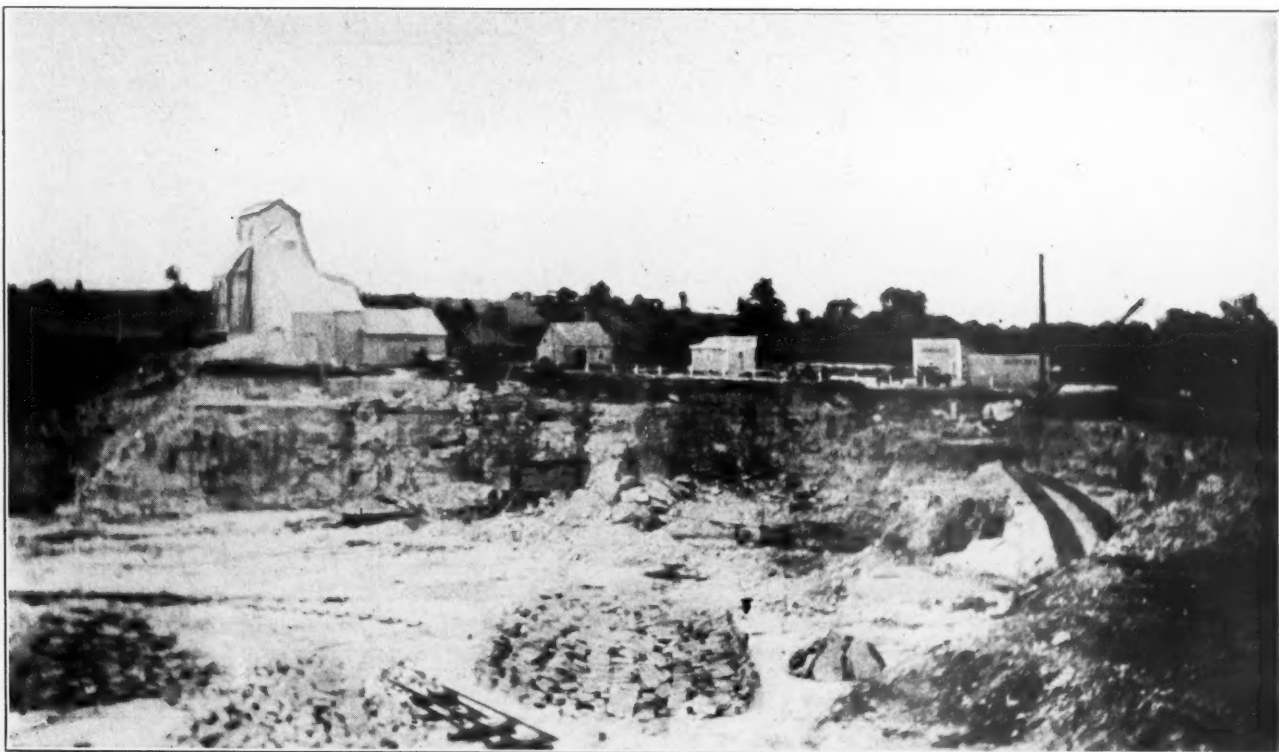
View of Quarry from Derrick Number 2, Looking Toward Crusher Buildings
